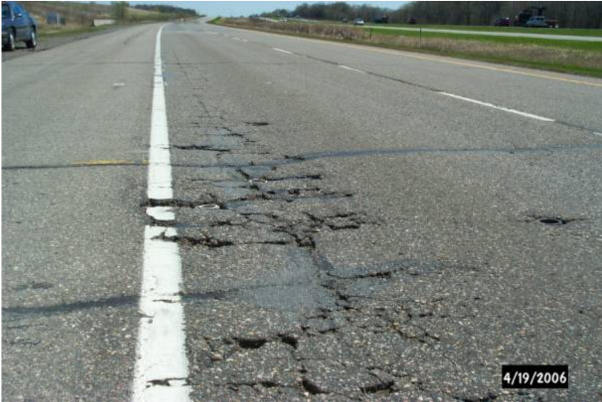
**Figure 2. Cell 1 Pavement Condition**
