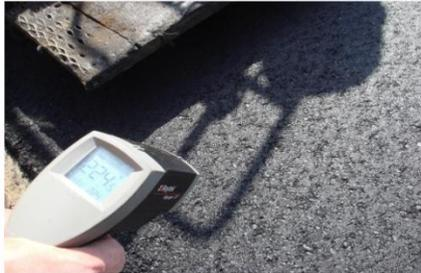
Warm mix asphalt (WMA) is a general term describing the use of any additive or technology that allows for lower asphalt plant mixing temperatures. Developed in Europe, WMA was brought to the United States in 2004 and has since gained widespread use around the country. Environmental benefits experienced with WMA include reduced emissions, fumes, and odors. With a cooler work environment enabled by WMA technology, reduced production temperatures add up to energy savings. The
